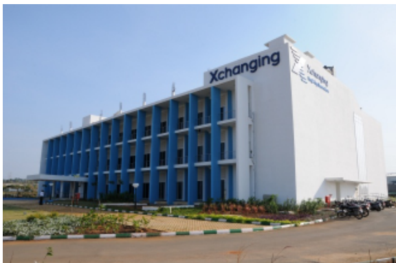
Figure 13: The completed building (from northwest)
