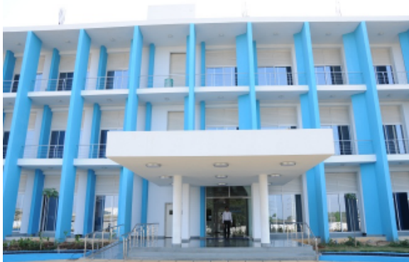
Figure 12: The north façade and building entrance.
